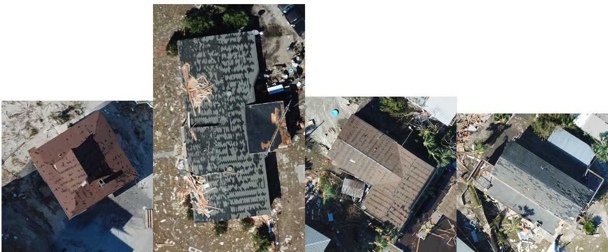
Figure 8. Example buildings labeled 'minor damage'.
