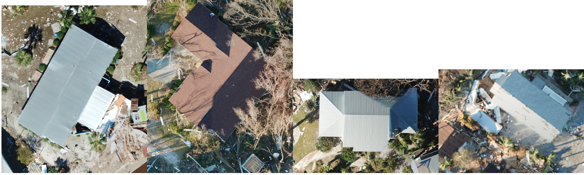
Figure 7. Example buildings labeled 'no damage'.
